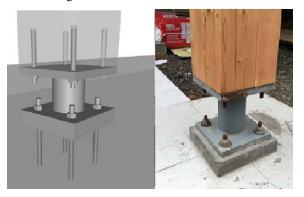
Figure 3: Typical connection ground floor; Left: 3D model (Courtesy CADMakers), Right: Picture from mock-up
