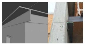
Figure 4: Typical connection between core and CLT floor; Left: 3D model (Courtesy CADMakers), Right: Picture
