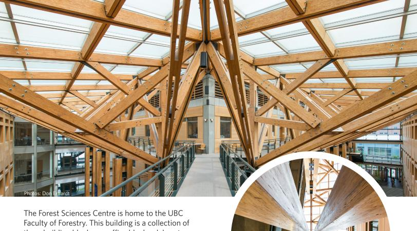
three building blocks: an office block, a laboratory, and a wood processing centre, all of which surround a large central atrium. The atrium is known for its 13-meter-tall parallel strand lumber (PSL) columns and a branch-like system of trusses, used to support the skylight roof. The columns are connected to the branches using hybrid steel-to-wood connections. The atrium walls are lined with Douglas-fir boards and
